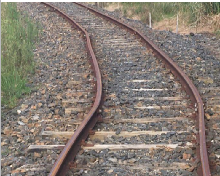
Left: track issues after the recent events (P. Cairncross). Right: a clear view of the line, with the challenges of keeping the vegetation under control! (C. Mann)
