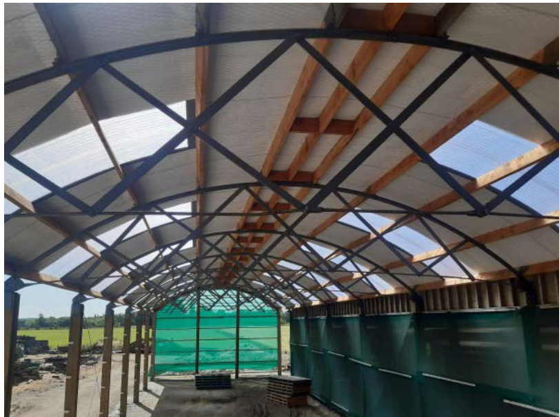
Inside the Gulley Building
