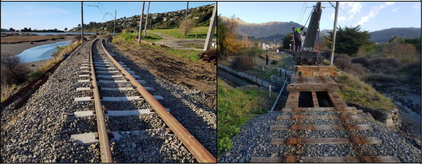
Above Left: 50kg rail placed on new concrete sleepers. Right Removing sleepers off the bridge beams.
