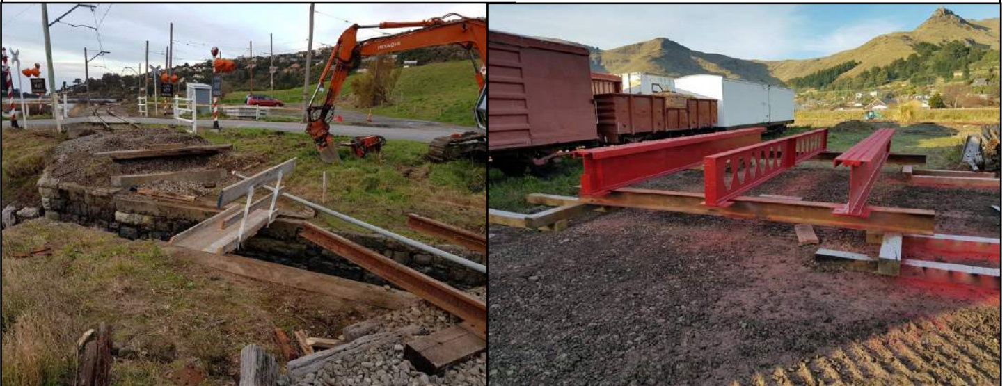
Above Left: Temporary access bridge in place. Some work to do on the bridge abutments and surrounding areas, before the bridge goes back in. Bridge rebuilding includes ballast guards to be extended and new wing walls to be constructed. Right: Bridge beams have been painted.
