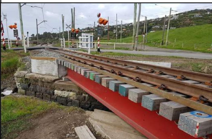
Above: The four tasks of the project: painted bridge beams, with extended wing walls, the re-laid track, the new asphalt level crossing and the soon to be commissioned level crossing alarms. Photo: Peter Jenkinson
