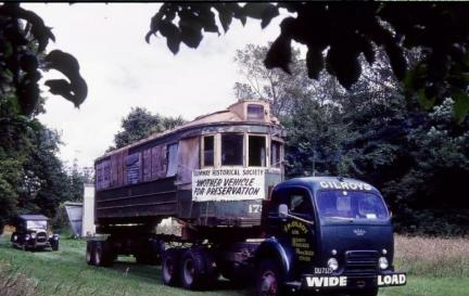
The recovery of 'Brill' 178 from its old home at the Milford Huts: what started out as a tidy holiday cabin soon came down to reveal a somewhat complete tram body, still painted in its final CTB livery. Fitted neatly onto Gilroy's transporter, and lifted with the help of a mobile crane from the Timaru Harbour Board, 178 began its journey back to Christchurch in January 1967.
