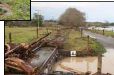
Photos from left: Evidence that the water covered our railway tracks leaving the tree debris. Bridge over Tirohanga Stream. Railway track had obviously been underwater. Clear up can only happen when waters recede, and track stability has been checked. Another section of track in Taumarere area
