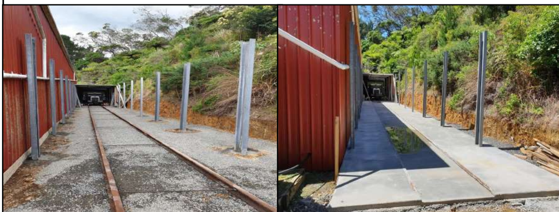
Left: Progress on the wood-work shop "lean-to" showing the rails in place and posts concreted in. Photos: I. Jenner.
