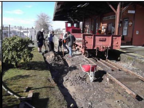
Bill noble in charge of our track gang took after yesterday's working bee up at the Pleasant Point railway station. The railway track in front of the station is the only part of the Fairlie branch line that is still in use. the rest of our track has come from many sources. The veranda railway line that supports over the station platform are also part of the track the train ran over. Photos: Bryan Blanchard.
