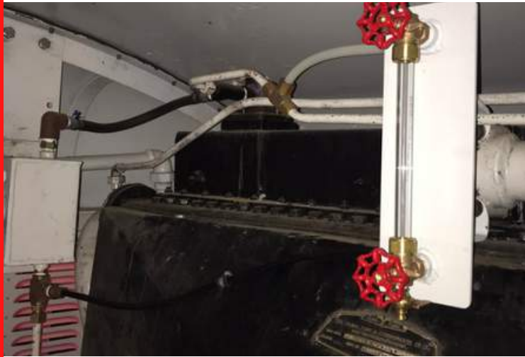
Left: Sight glass in place in radiator room. Right: New wiring being run for pressure switches. Photos: DTG Facebook
