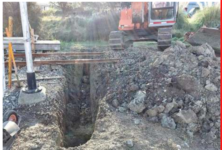
Left: Tr156 and work train. Refurbishing the track sets for the Valley Station loop. Right: Trenching under the Branch Line track for the new drainage pipe. Photos: Branchlines
