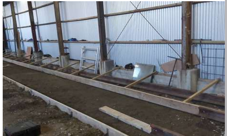
Left: a near 40m long concrete track beam being prepared for fixing rails on the East side in the long No 2 Railcar Shed. Right: West side boxing prep. Photos: Facebook
