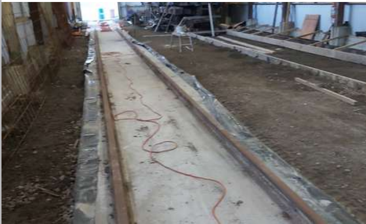
Left: a near 40m long concrete track beam being prepared for fixing rails on the East side in the long No 2 Railcar Shed. Right: West side boxing prep. Photos: Facebook
