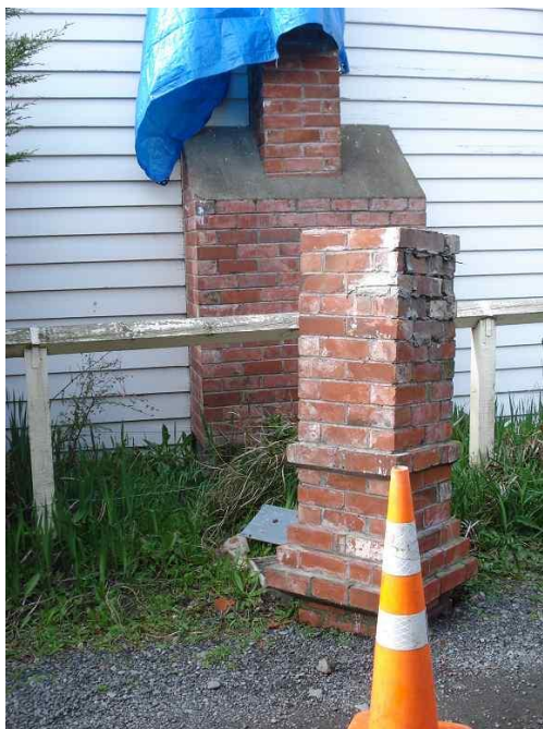
Ferrymead School Chimney Photo : Flugel
