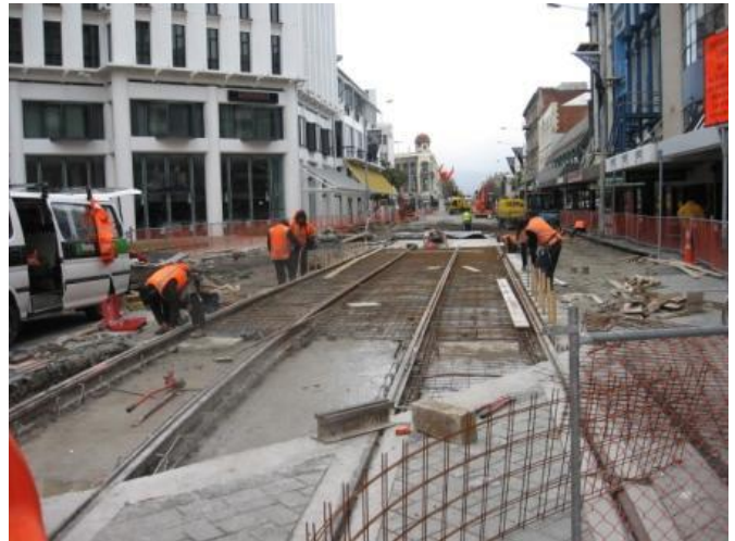
Christchurch Tramway Extension, High Street
