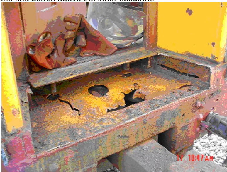
Severely corroded shearplate and collision posts (riveted construction)
