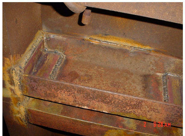
Welded replacement for a riveted transom
