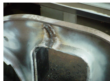
Typical repair to crack in horn opening
